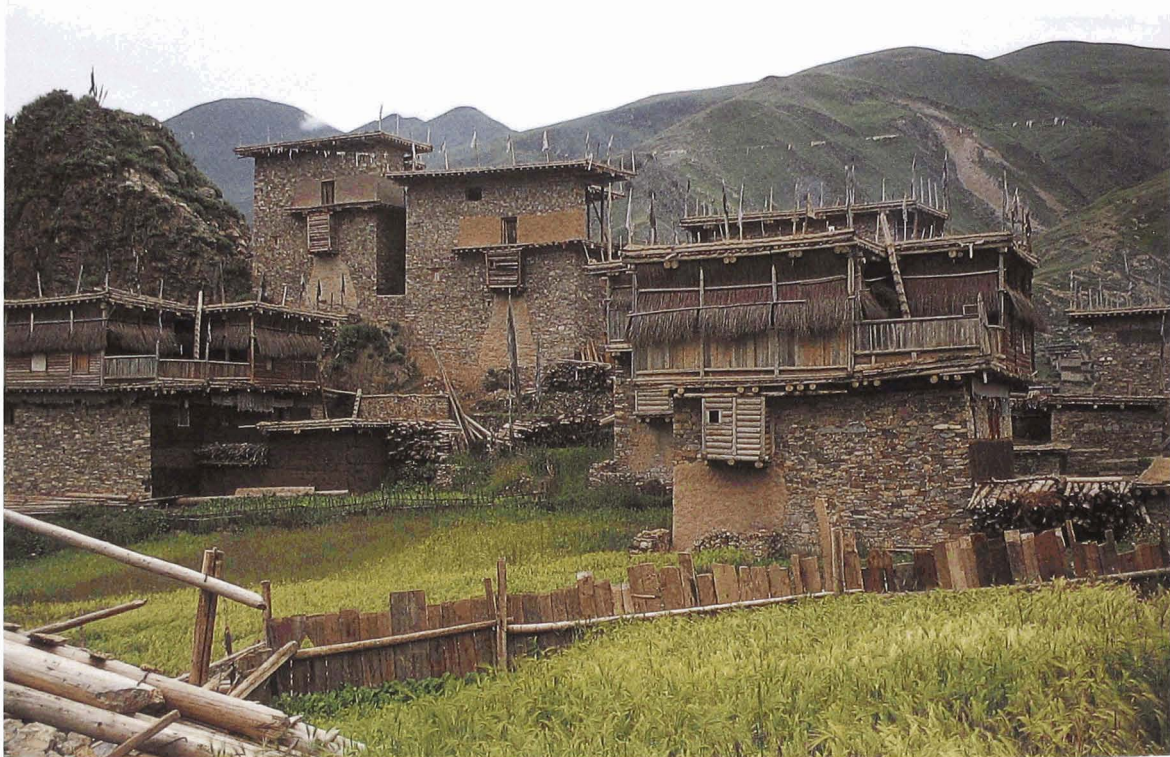
174. The farmhouses have either two or three floors, with wooden overhanging balconies, and are topped by enormous open lofts used to store and dry the corn.
