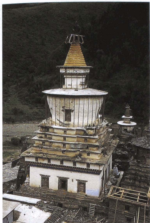
116. With a height of 42 m and a ground space of 484 square metres the chörten of 1910 belongs to the largest examples of this architectural type in the Tibetan realm.
